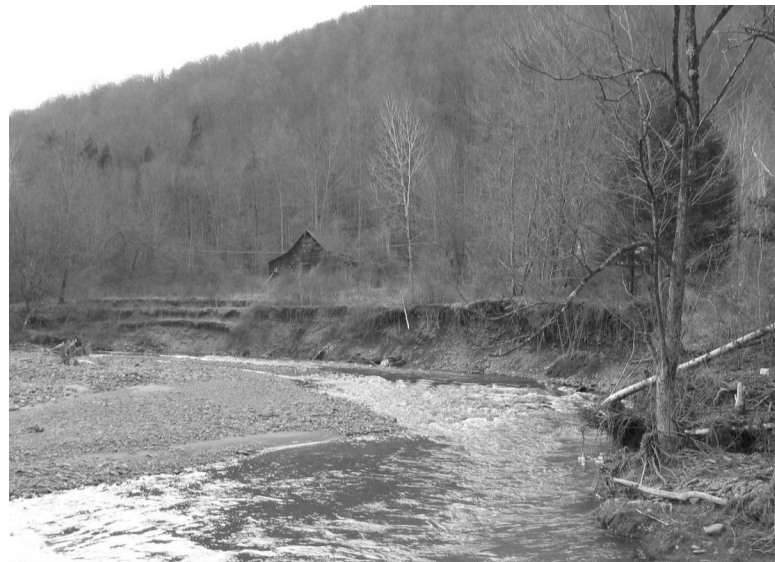
Figure 15. View upstream toward actively retreating streambank with rotational failure scarps exposed in adjacent terrace (photo courtesy DEP, 2006).
