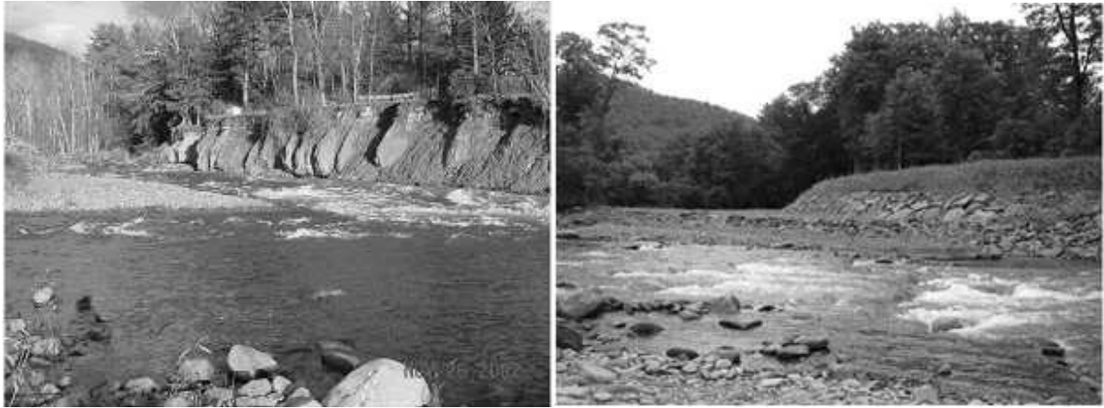
Figure 11. Esopus Creek at Woodward Valley restoration site before (left) and after (right) restoration project. Post-project photo taken July 13, 2004, approximately 9 months after construction, but before major flood in April 2005. From Barnet, 2004.
